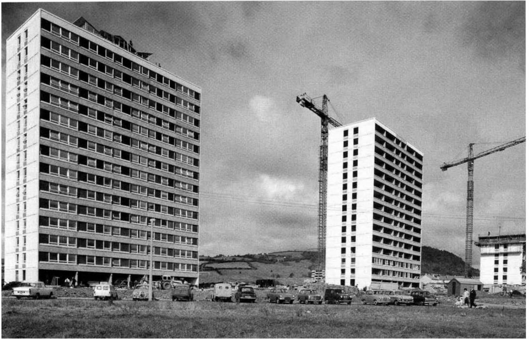
29.4. NIHT's Rathcoole Development 14 (four 15-storey Sectra blocks); photographed under construction in 1965.
