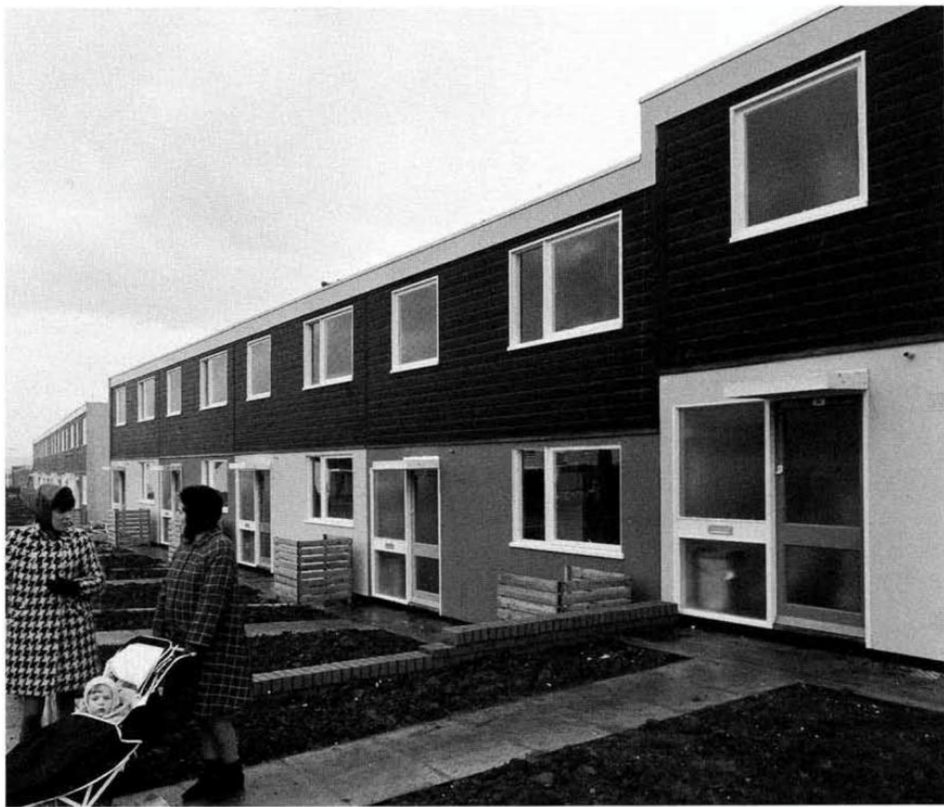
29.5. Prototype two-storey Sectra terraces built by NIHT at Monkstown, Newtownabbey: photographed following completion in 1970. The dwellings, each one Sectra tunnel wide, were timber-clad (the ground floor being coated with SBD Stonepaint). ( Belfast Newsletter )
